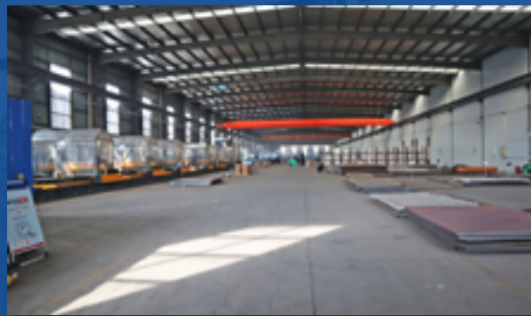
Overlay wear plate workshop
